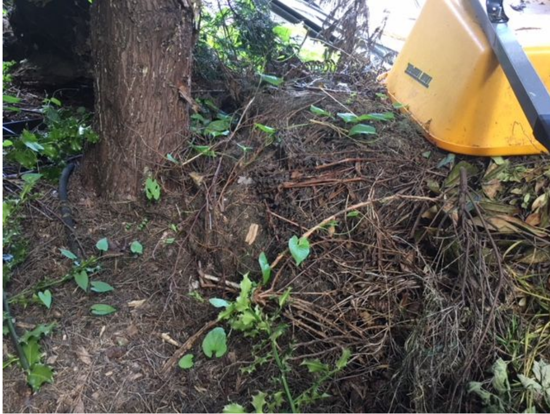
Photo of tree #2, Western Red Cedar, with fill material placed over root zone.
